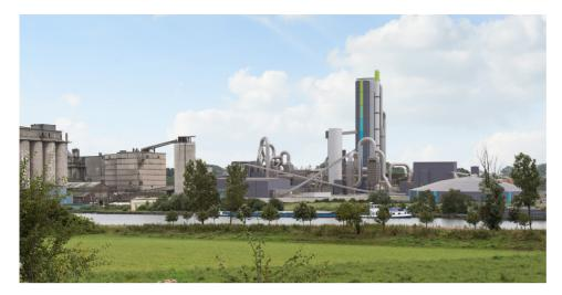
Innovative new air-oxyfuel switchable cement kiln to facilitate the capture and purification of CO2, for geological storage in the North Sea and/or for an innovative e-fuel production scheme.
